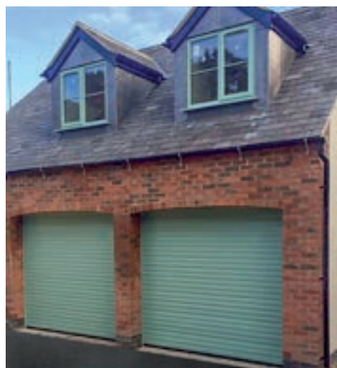
Garage under a bedroom?
